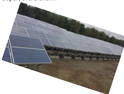
Above and below are photos of the landfill ground ballasted system.
