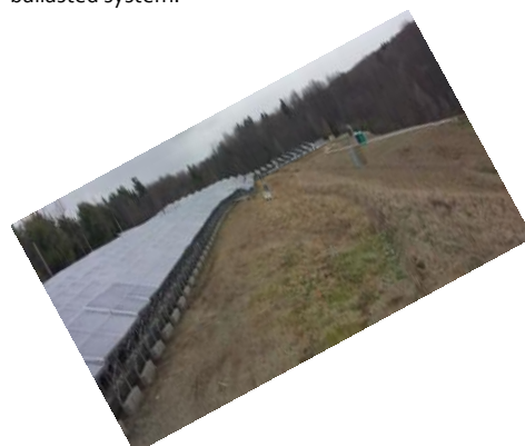
Above and below are photos of the landfill ground ballasted system.
